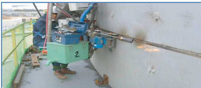
Horizontal Automatic Welding
