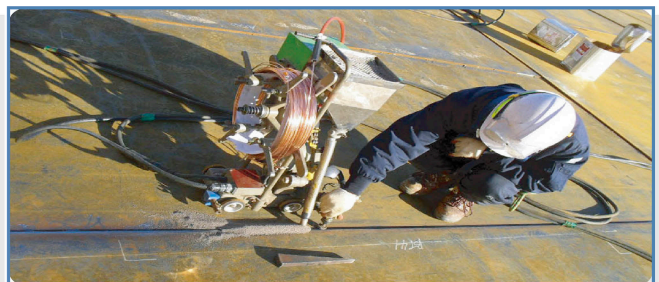
Bottom Automatic Welding
