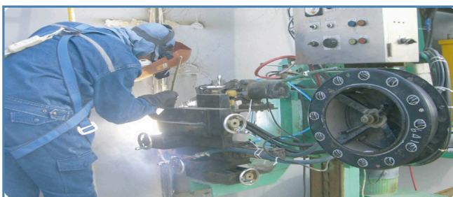
Vertical Automatic Welding
