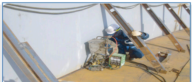
Corner Automatic Welding
